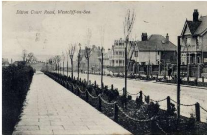
Ditton Court Road looking south showing the planting and post and chain edging
