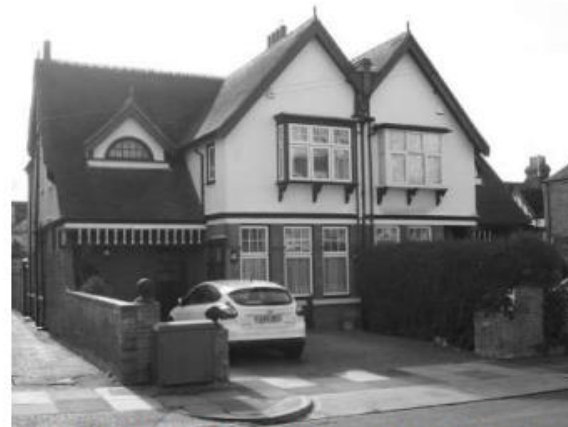
42 Preston Road: Edwardian semi-detached with fine roof form and paired gables and bracketed bay windows and decorative balustraded porch canopy. Simple lunette dormer window (referencing DCR). Familiar Edwardian window design of multi-pane over single pane (albeit modern replacements)
