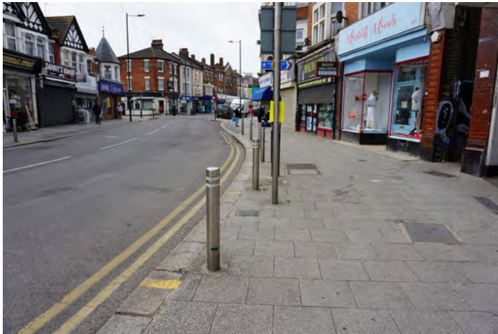
Stainless steel bollards, square paving, granite kerb stones and absence of greenery
