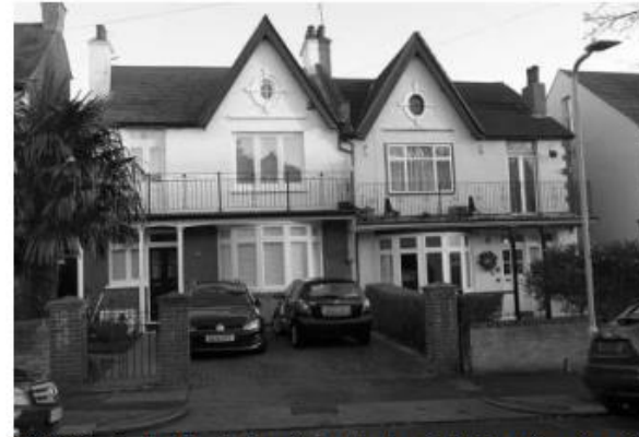
26-24 Cossington Road: A semi-detached pair of Edwardian villas with centrally paired gables with bull's eye windows, full width balconies creating entrance porches and ground floor bay windows
