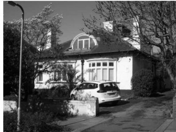
46 Ditton Court Road: an Edwardian bungalow with bay windows, lunette window and tapering chimney stacks
