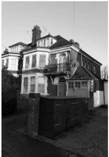
19 Ditton Court Road: two substantial semi-detached houses with embellished bay windows and arched doorways
