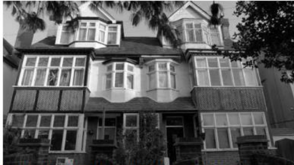
69/67 & 71/73 Ditton Court Road: Two of an impressive row of Edwardian houses built as maisonettes on the east side of the road with dominant bay and dormer windows, echoing others in the road
