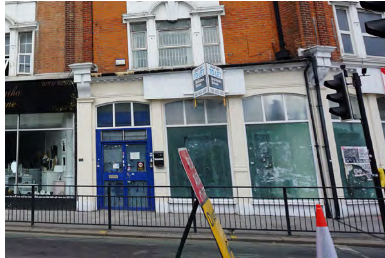
Shop front mainly surviving on No.209 Hamlet Court Road
