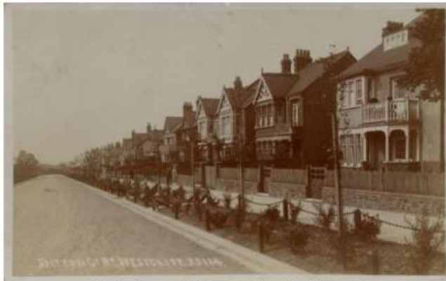
A further image of Ditton Court Road looking south
