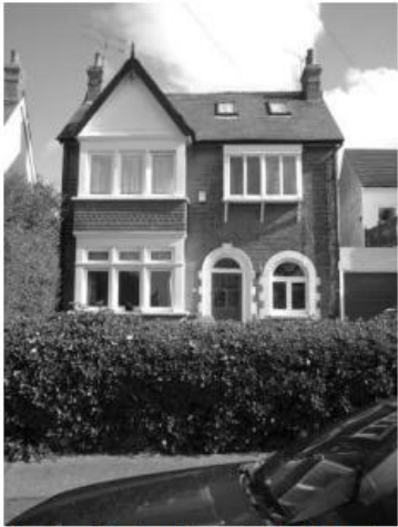
18 Ditton Court Road: a detached villa with emphasised arched entrance. Note repeat of door type to previous image
