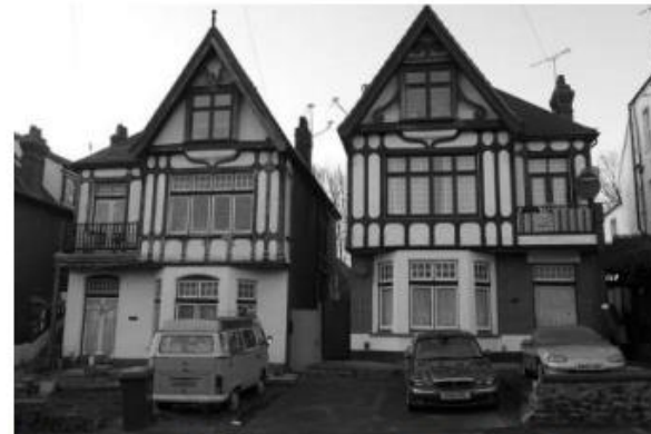
7-9 Cossington Road: A dramatic pair of half-timbered detached Edwardian villas with heavy timber detailing. No. 7 is not in good repair but is repairable. No. 7 appears to retain most of its original windows as multi-pane lights over Casements. At ground floor are bay windows
