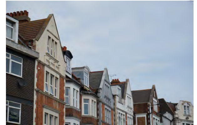
Varied and interesting roofline on Hamlet Court Road
