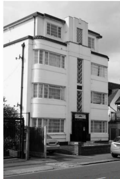
Sunray House: This is a white rendered Art Deco block of flats with two curve fronted bays with what appears to be the original horizontal Crittal windows intact and a bold central bay with chevron glazed vertical light, contrasting black entrance with coloured light motive. The top floor is a modern addition.
