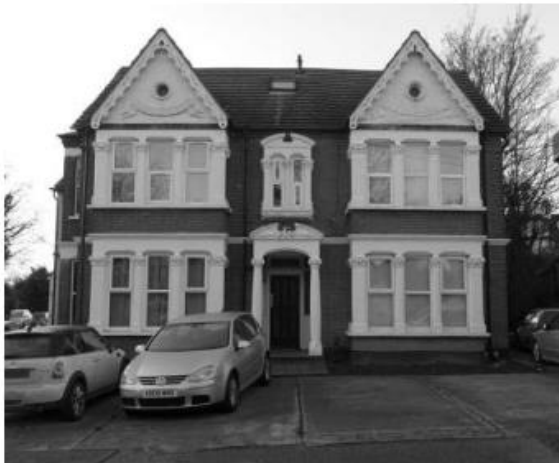
1 Cossington Road: A substantial red brick double fronted villa with identical twin bays with decorative gables including ornamental barge boards, bull's eye windows and insignia swags. Ornamental column entrance with segmental arch pediment and similarly decorated window above
