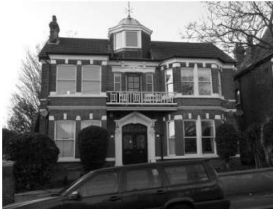
3 Cossington Road: A substantial red brick double fronted villa with square and angled bay windows to either side, a framed, arched and pediment entrance, balcony and decorative tripartite window above, all topped with a turret cupola
