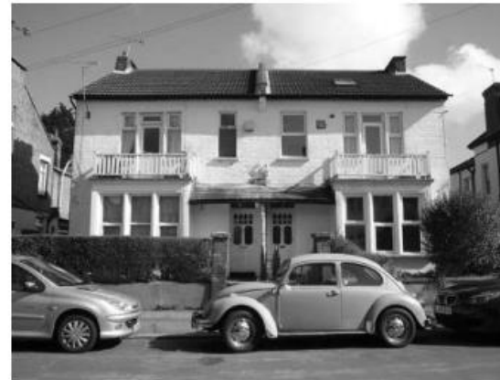
8-10 Ditton Court Road: two semi-detached houses with original balconies and front doors
