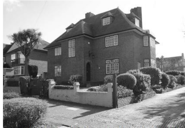
27 Ditton Court Road: a substantial house c.1938 recalling the Arts & Crafts of Voysey, Mackintosh, Lutyens and Baillie Scott
