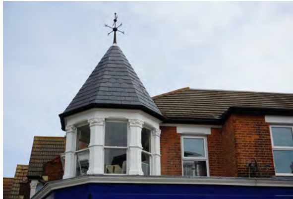
Patterned slate tiles to the turret of No.170-172, with red clay tiles to the right and examples of unsympathetic concrete tiles to the left
