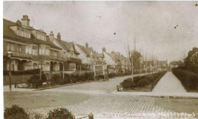
Ditton Court Road looking north from Canewdon Road. Note the post and chain edging widely used at Hampstead Garden Suburb
