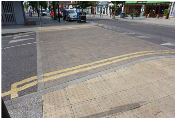
Tactile paving and brick setts used at pedestrian crossings points
