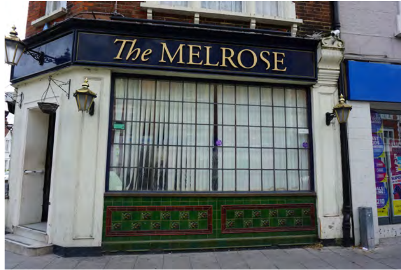
The Melrose public house, with coloured glazed tiles to the stall riser, leaded glazing, fascia board proportionate to the flanking corbels and pilasters
