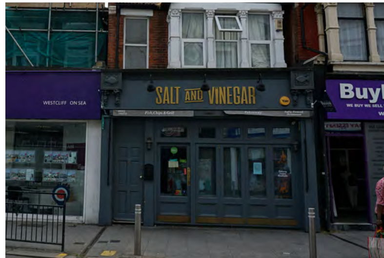
No.186, 'Salt and Vinegar', a modern shop front in an appropriate traditional design
