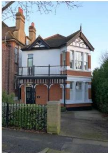
32 Cossington Road: A detached corner property with a dominant corner facing bay and half-timbered gable. A second decorated gablet elevates the flank which also has a decorative balcony and entry porch
